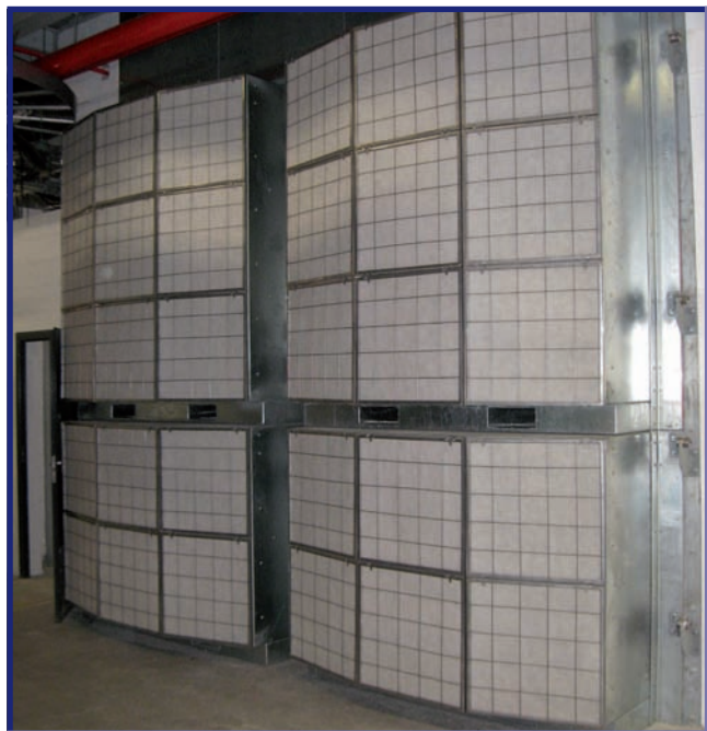
The removable filter wall in front of the attenuators.
