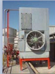
Single Cell Forced Draft with Axial Fan
