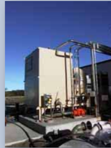
Single & Multiple Cell Forced Draft With Low Noise Centrifugal Fans
