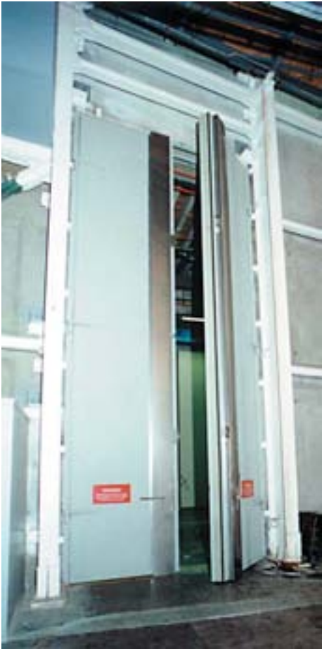
45dB, two hour fire doors at Auckland's AOTEA Centre
