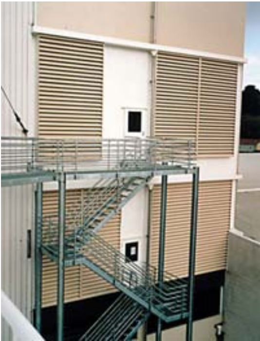
Windsor louvres in powder coated aluminium on a dairy factory plantroom
